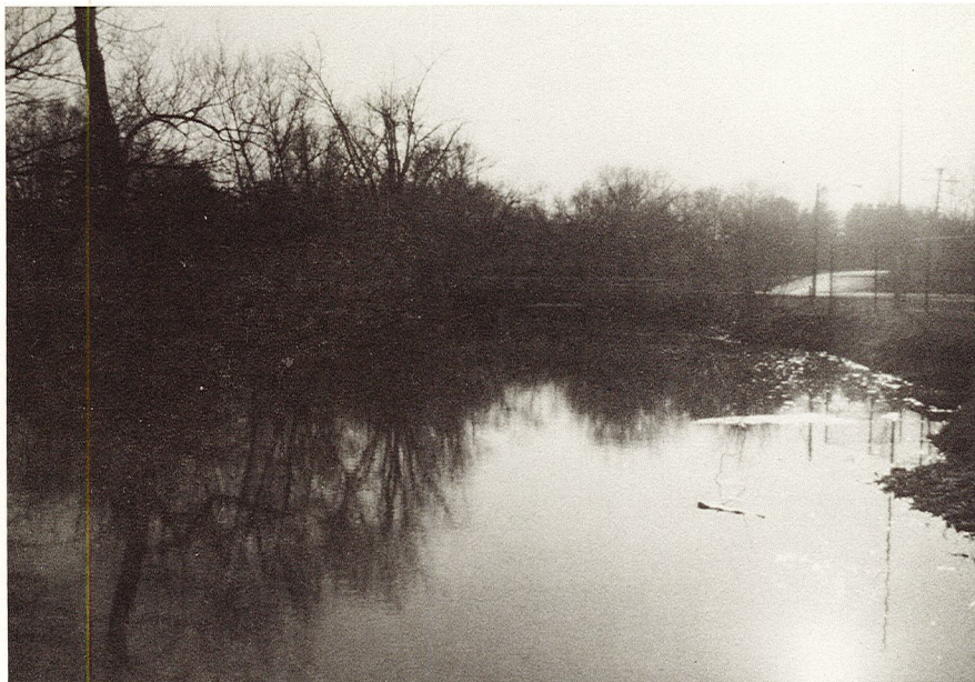
CENTERVILLE CREEK HIGHWAY LS BRIDGE FROM LAKE MICHIGAN SHORELINE, PRESENT VIEW
