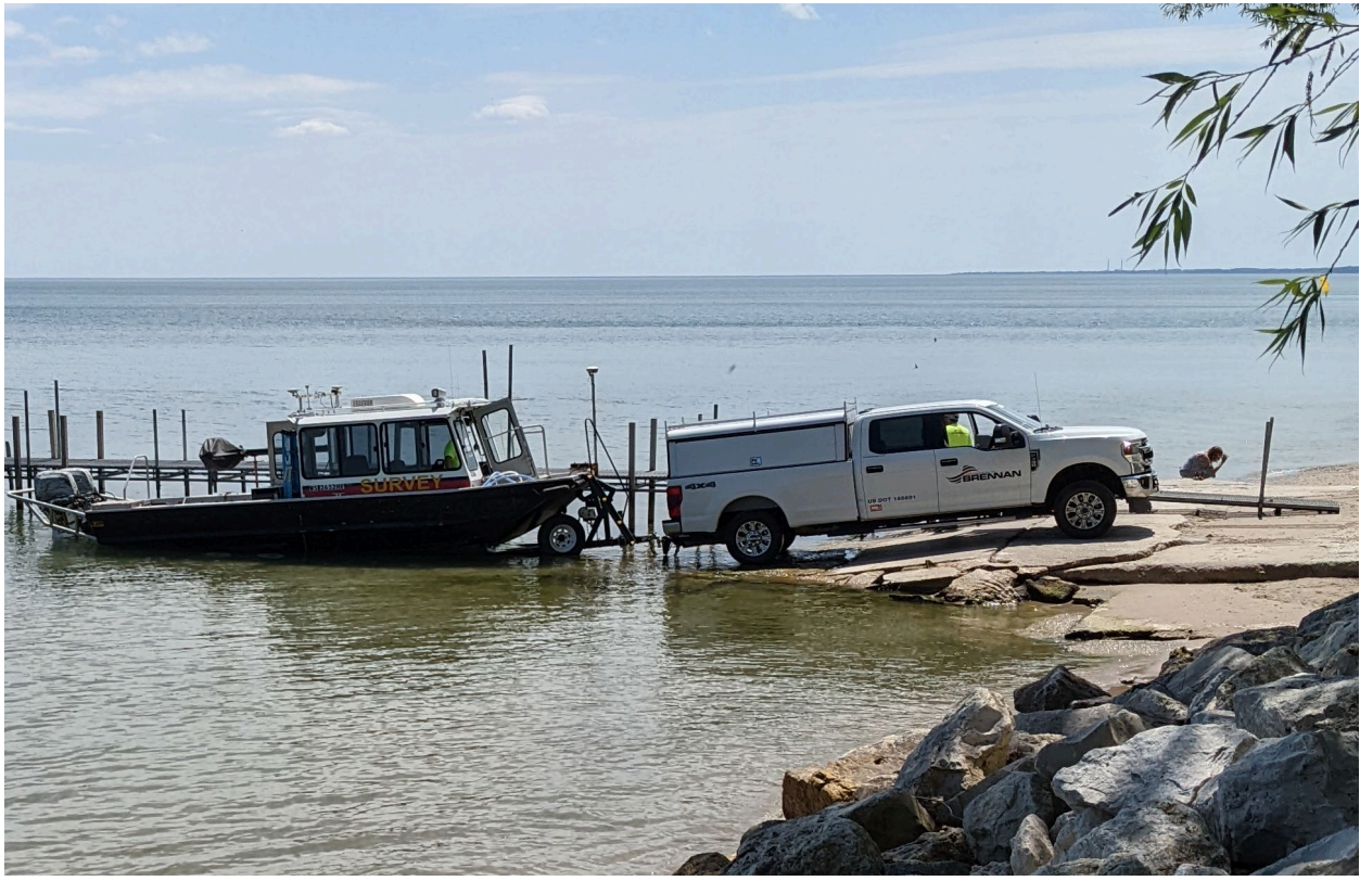
Figure 2.1: Existing Concrete Boat Launch Ramp (Photo 1 – Baird, 2022)
