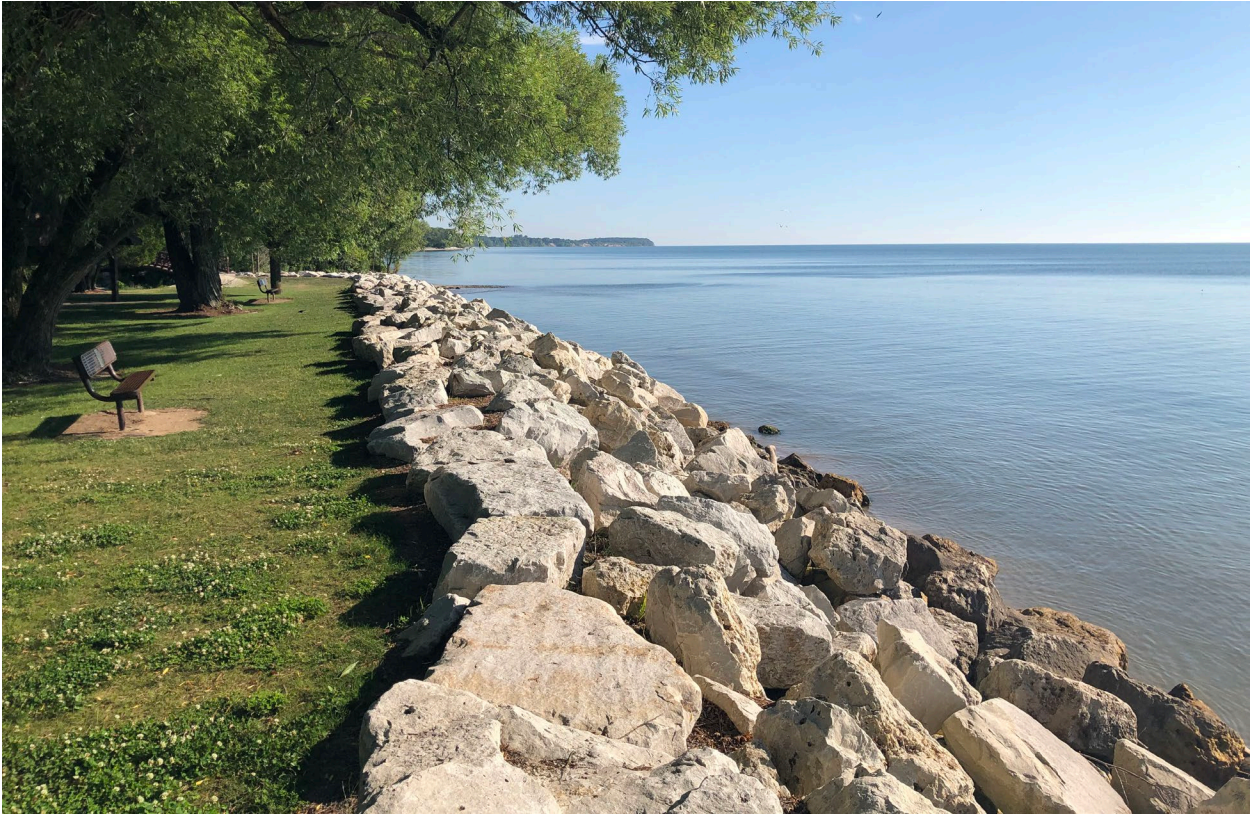
Figure 2.4: Shoreline Revetment (Baird, 2022)
