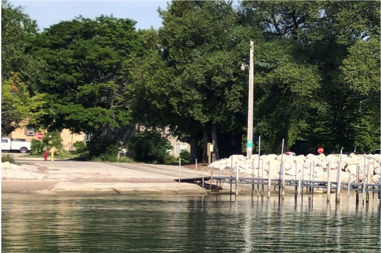
Figure 2.2: Existing Concrete Boat Launch (Photo 2 – Baird, 2022)
